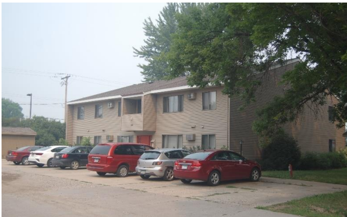
5 th Street Apartments
